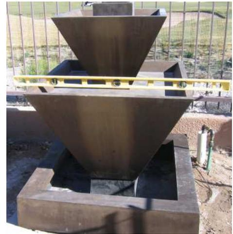
After filling the fountain with water and running the water we noticed the water flow was not exactly even all the way around so we adjusted our shims accordingly until the water flow was even. Afterward we trimmed our shims so they would not be visible. Trimming these plastic shims is just a matter of snapping them off as close to the base as possible.
