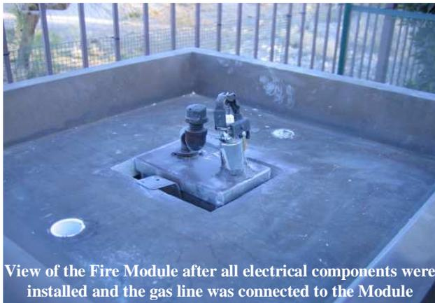
View of the Fire Module after all electrical components were installed and the gas line was connected to the Module
