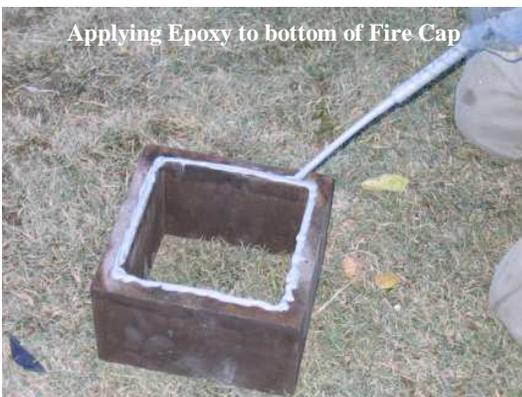
Applying Epoxy to bottom of Fire Cap
